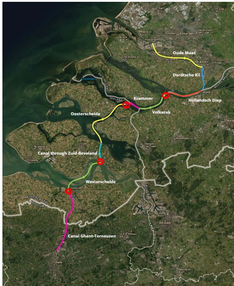
Figure 3. Big Picture Overview of an IWW route between Rotterdam and Ghent (©AEGIS [2])
